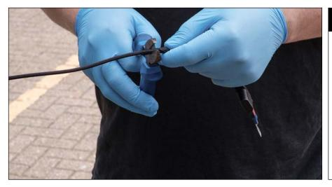
Extend the battery connection wire from the supplied wiring kit by first cutting off the fuse holder and ring terminal.
